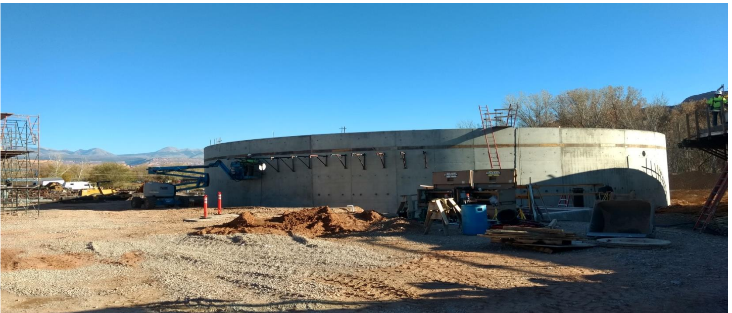
Moab Sequencing Batch Reactor Tank Nov 2017
