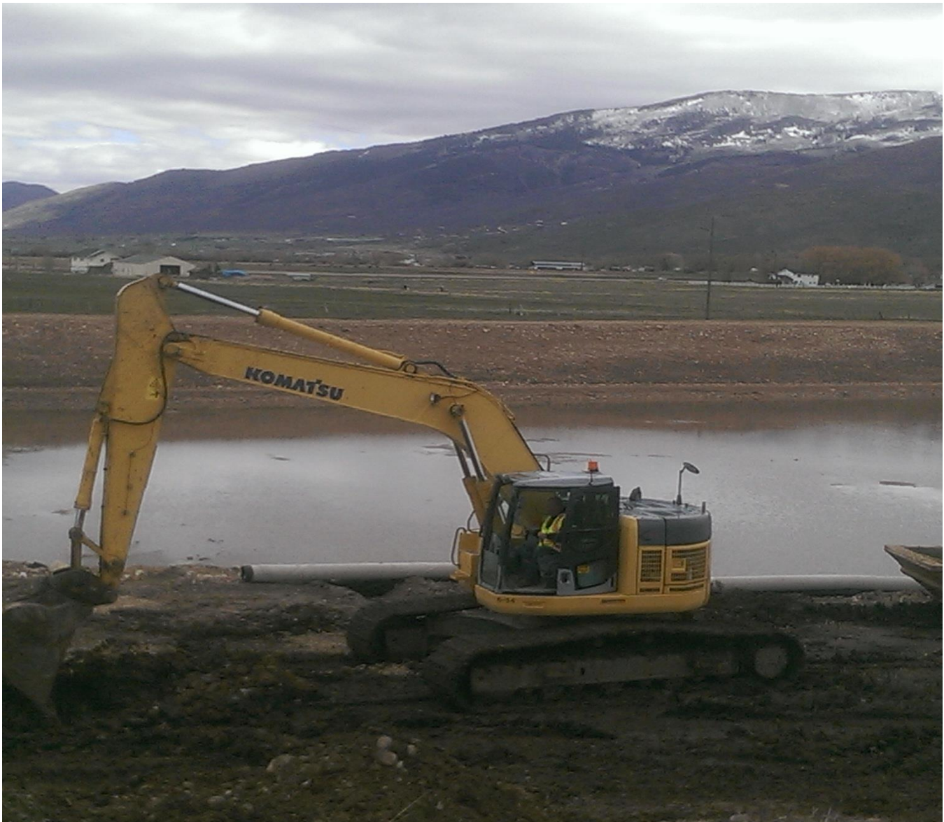
Construction on the Francis City Project
