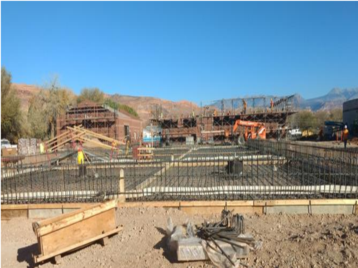
Moab Construction Nov 2017
