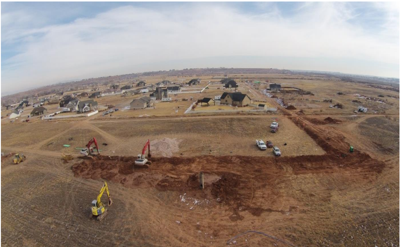
City of Roosevelt Arial View of Sewer Project Construction
